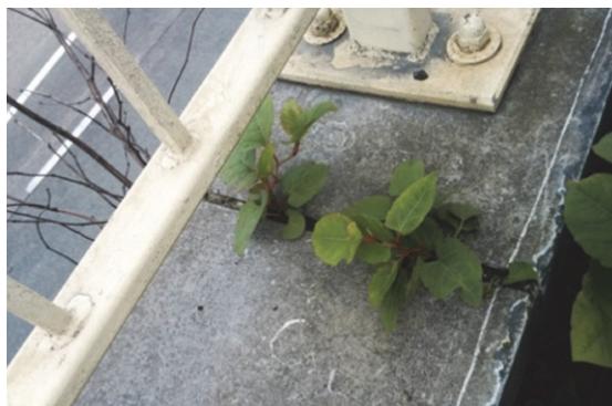
Figure 19. Japanese knotweed growing in cracks and damaging bridges (left) and railway platforms (right). Source: Thoonen & Willems (2018)
